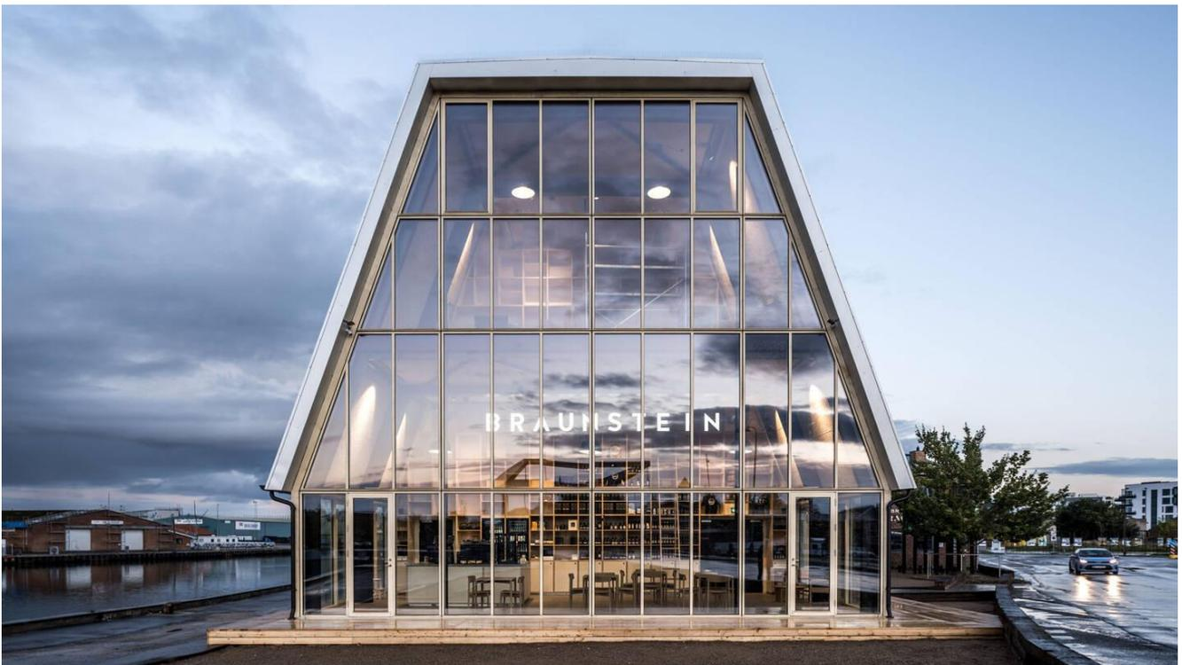
The building uses as few materials as possible, among them Junckers Textured Oak two-strip hardwood flooring. The structure is based on simple tectonic principles, completed with mechanical joints only. As far as possible, building materials used in the construction are not mixed, allowing for removal without contamination and reducing the volume of waste considerably in comparison to similar constructions.
